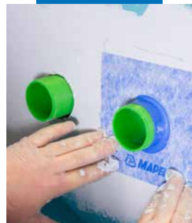
Mapei VR Collar installed in Mapegum WPS
