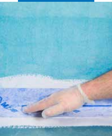
Installing Mapei ST sealing tape using Mapegum WPS, floor/wall transition
