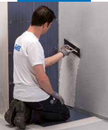
Application of tile adhesive
