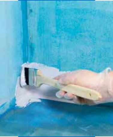
Installation of Mapei IC/EC corner gasket using Mapegum WPS
