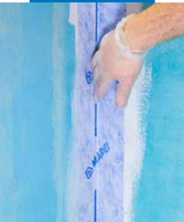
Installing Mapei ST sealing tape using Mapegum WPS, wall
