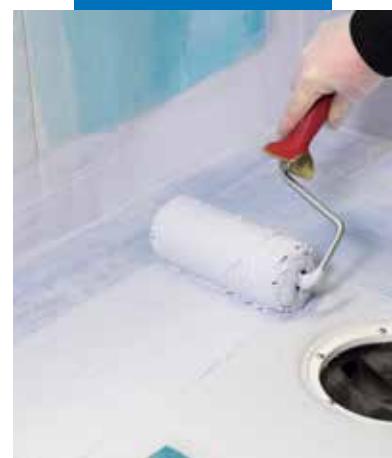
Application of Mapegum WPS membrane with e.g. a roller
