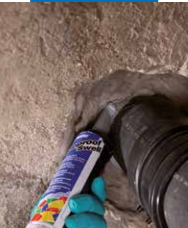
Through element sealed using Mapeproof Swell
