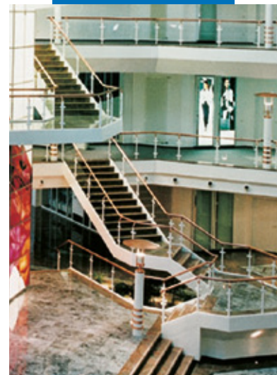
An example of an installation of ceramic or marble on a metal structure (stairs)
