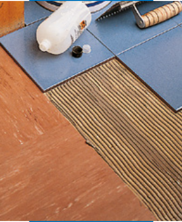
Laying on an old PVC floor
