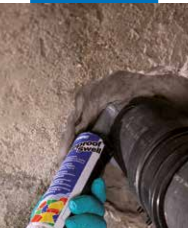
Through element sealed using Mapeproof Swell
