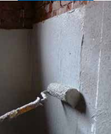
Application of Mapelastic Foundation by roller on a substrate evened out using Planitop HDM Maxi
