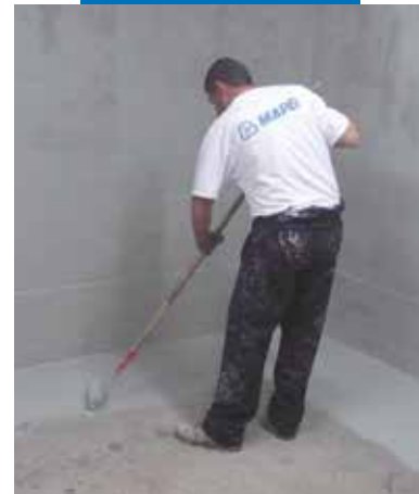
Mapelastic Foundation spread on by roller to waterproof against water in negative pressure
