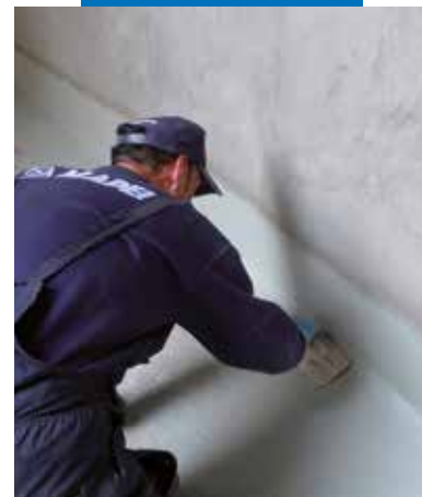
Mapelastic Foundation spread on by trowel to waterproof against water in negative pressure
