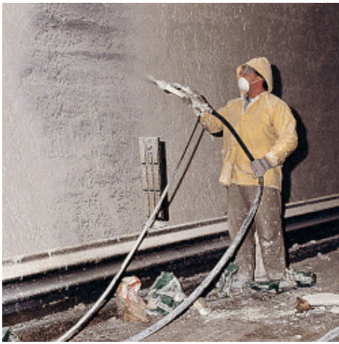
Application of white Planiseal 88 by spray gun in highway tunnel
