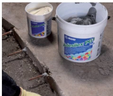
Fixing reinforcement rods for the dowelling in place using Adesilex PG1
