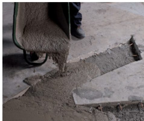
Application of Mapegrout SV Fiber in the area under repair
