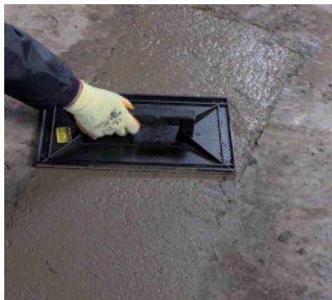
Tamping Mapegrout SV Fiber
