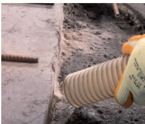
Removing dust with a vacuum cleaner
