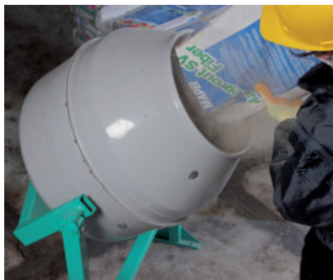
Preparation of the Mapegrout SV Fiber mix
