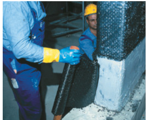
Application of MapeWrap onto the reinforced concrete element
