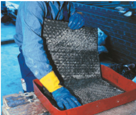
Manual impregnation of MapeWrap fabrics
