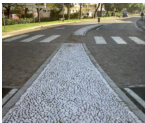
An example of a road with a central reservation in cobblestones
