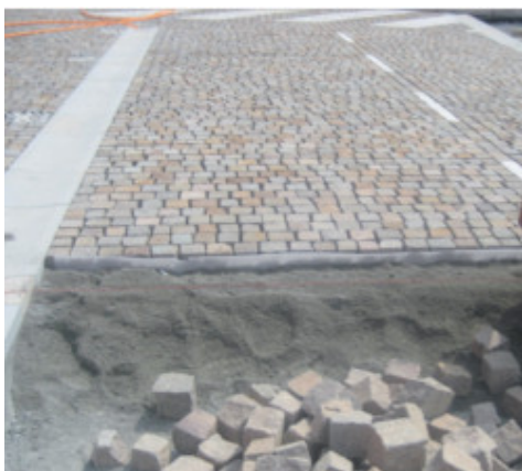
An example of an expansion joint
