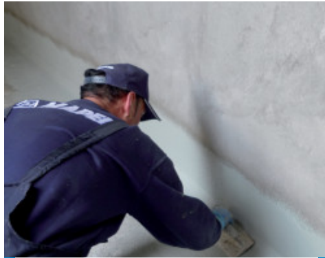
Mapelastastic Foundation spread on by trowel to waterproof against water in negative pressure
