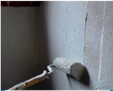
Application of Mapelastastic Foundation by roller on a substrate evened out using Planitop HDM Maxi
