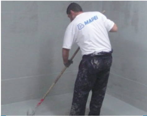
Mapelastastic Foundation spread on by roller to waterproof against water in negative pressure
