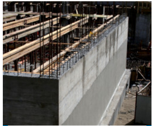
Retaining wall waterproofed after casting using Mapelastastic Foundation
