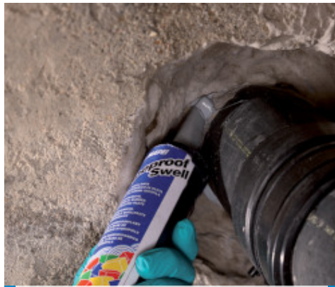
Through element sealed using Mapeproof Swell
