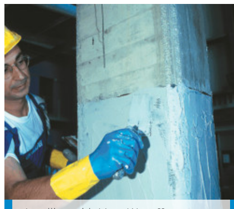
Levelling with MapeWrap 11 or MapeWrap 12
