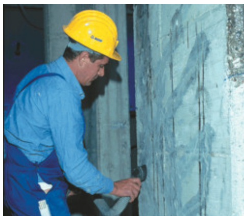
Preparing the substrate
