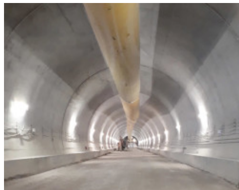
Example of final lining in a tunnel created using conventional tunnelling method
